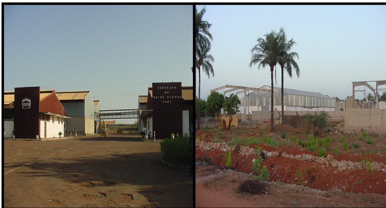
Fig. 11 – Zona Industrial de Alto de Bandim (CICER)
